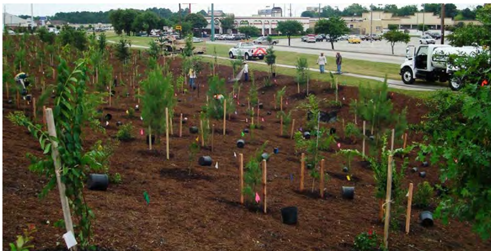
Figure 1.1: TxDOT forestation-style planting along I-69 in Houston
